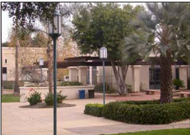
Frank Hall—Inefficient, unshielded fixture
