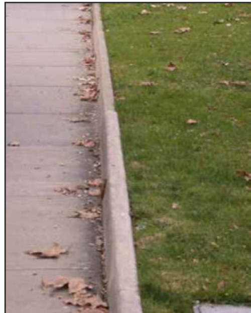
Curb and concrete walk, Bridges Hall of Music
