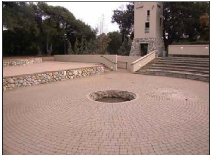
Permeable paving and stormwater infiltration Sontag Greek Theatre
