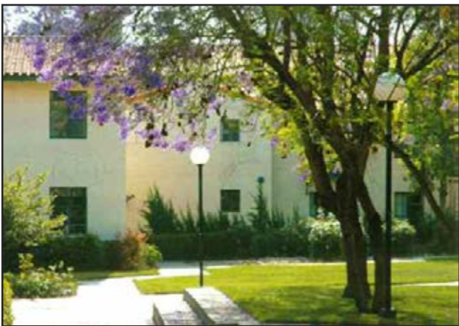
Lawry Court—Inefficient, unshielded fixture
