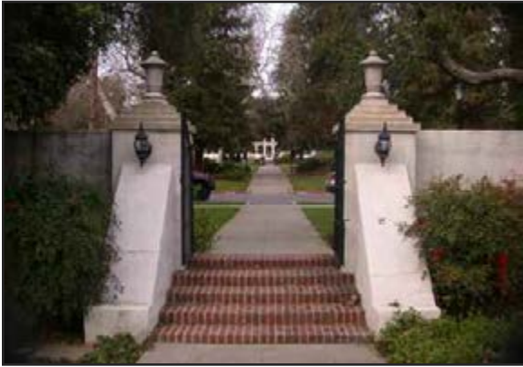
Smooth plaster finish walls, brick steps and concrete walk, Sumner Hall
