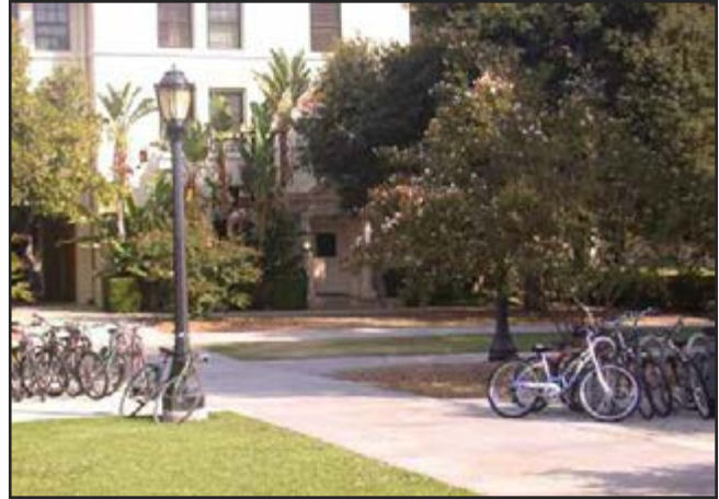
Campus standard fixture with non-standard, unshielded luminaire
