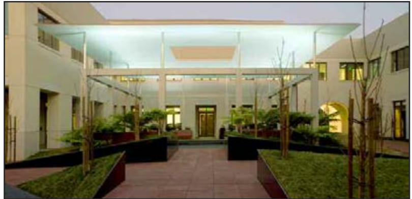
Integral color concrete paving with score line patterning Turrell Skyspace, Lincoln-Edmunds Courtyard
