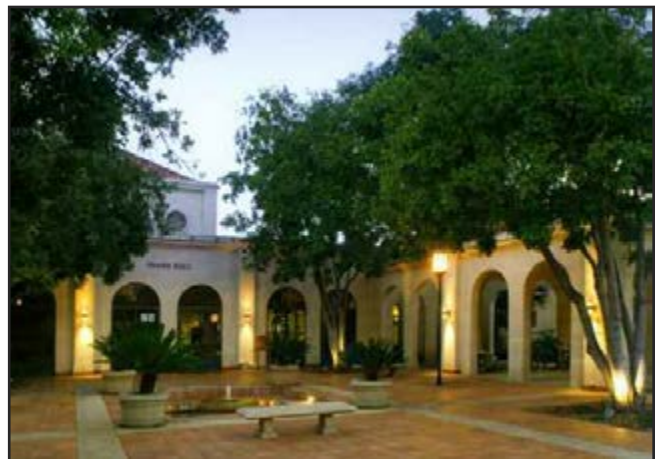
Frank Hall—Inefficient, unshielded fixture Frank Hall - Note the night time glare
