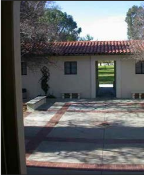
Concrete paving with terra cotta tile inlay, Clark I Dormitories
