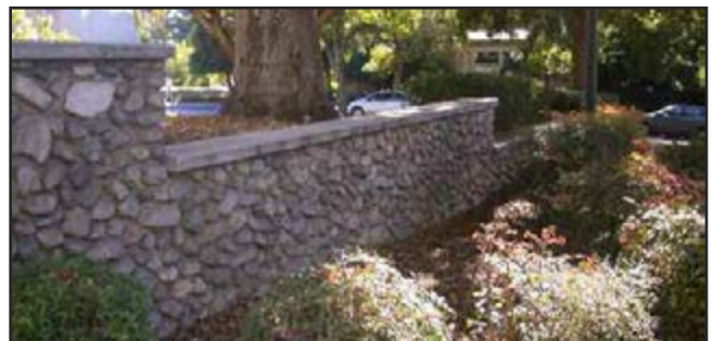
Historic stone walls, Carnegie Building
