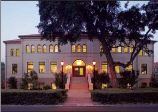
Pearson's Hall—Standard fixture with non-standard, unshielded luminaire (has since been replaced)
