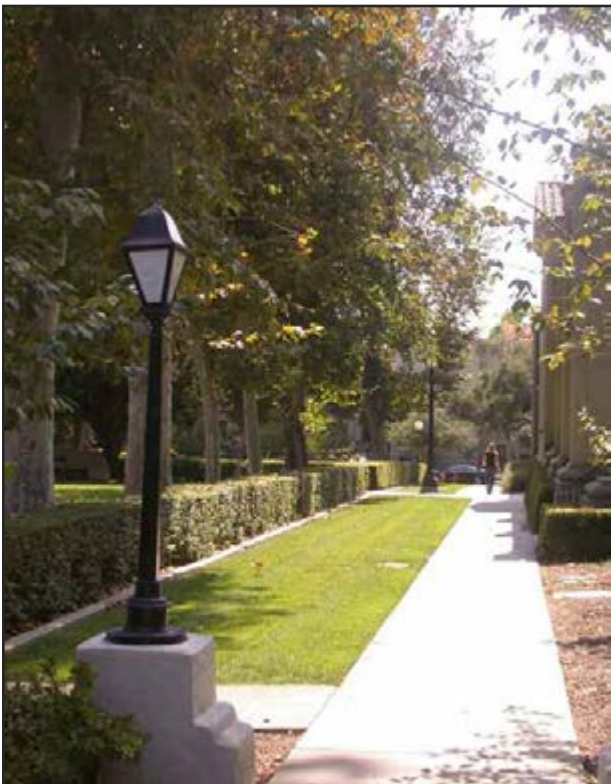
Memorial Court—Inefficient unshielded fixture
