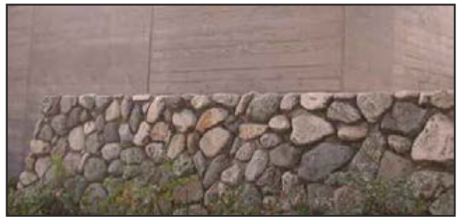
Board formed concrete wall, Local cobblestone wall, Pendleton Pool
