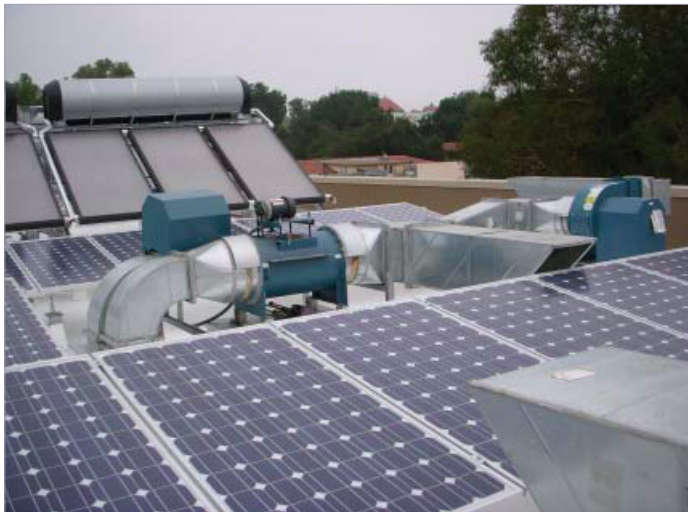
PHOTO: Sontag Residence Hall, rooftop solar panels
